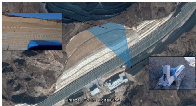
Figure 1. FastGBSAR-S deployment for monitoring a land slope next to a high-speed railway track.
