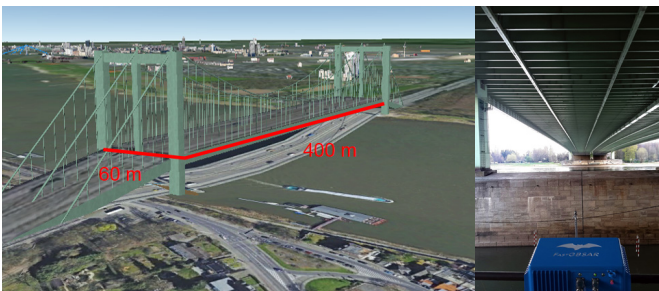
Figure 4: Highway bridge under observation.
